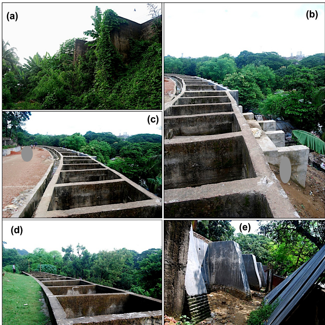
Figure 1.5. Reconstruction of the retention wall in Batali Hill, Chittagong. (b, c, d) top view and (a, e) bottom view. Source: Bayes Ahmed, field visit, September 2013 and July 2014.
