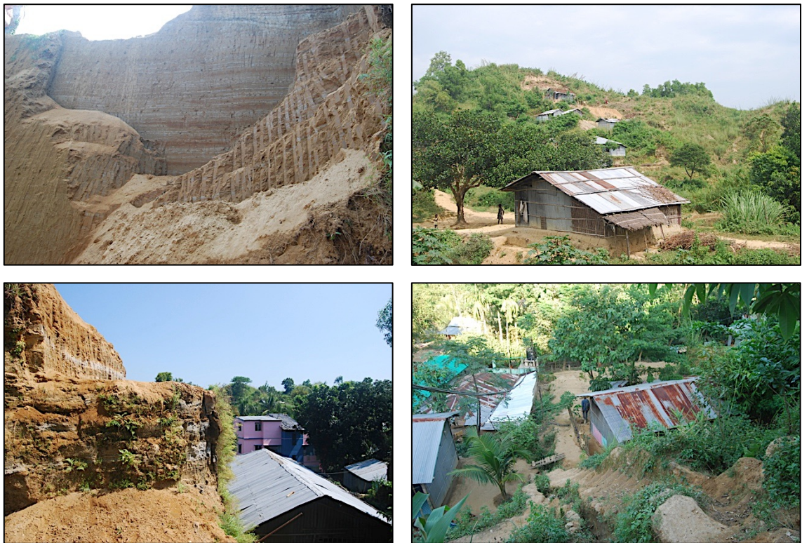
Figure 1.7. Systematic hill cutting to build residential houses in Cox's Bazar Municipality (CBM). Source: Bayes Ahmed, fieldwork, August to October 2014.
