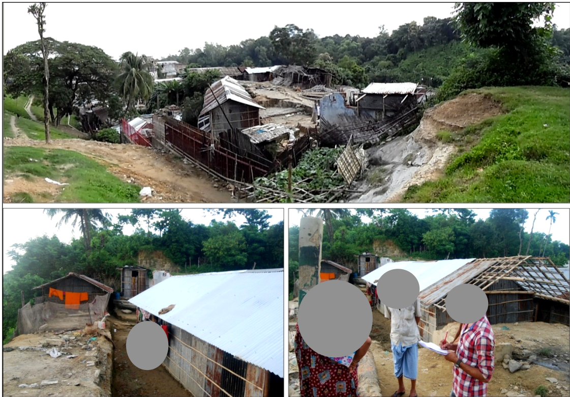
Figure 1.10. A cluster of highly vulnerable informal settlements at the top of Motijharna community was destroyed by the AC land office, Chittagong. Source: Bayes Ahmed, fieldwork, July 2014.
