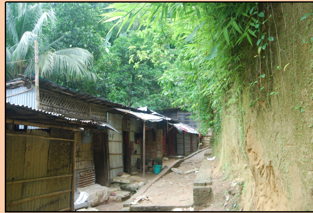
Figure: Semi-built, one storey Houses beside Hill
