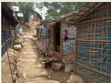
Figure 1a: Use of sandbags for the slope stabilization
