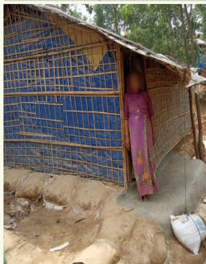
Figure 1b: Use of Tie Down Kits (TDKs) and bamboos to reinforce shelter
