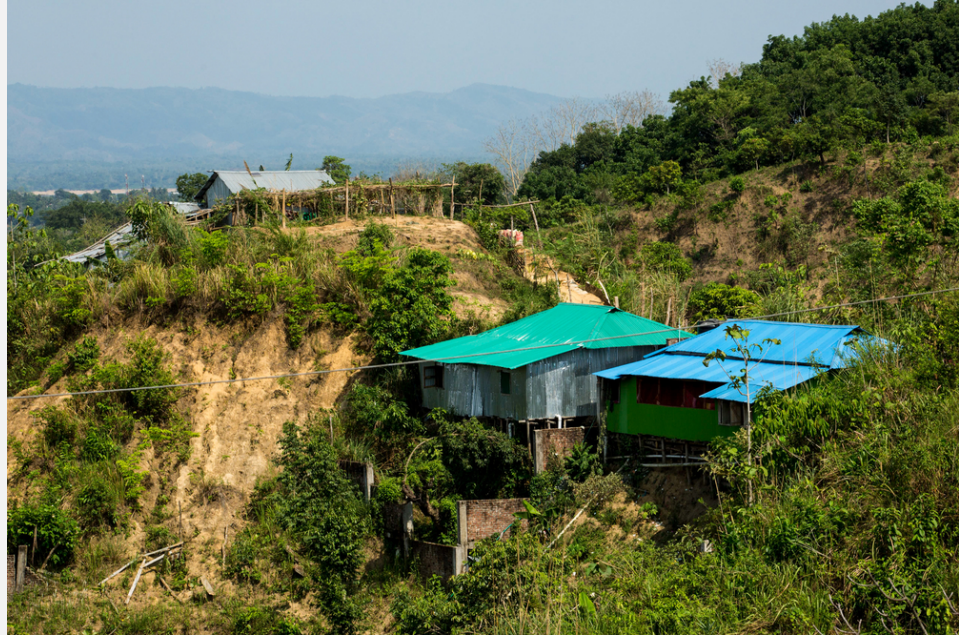
People in this settler community near Rangamati town have built their homes against parts of a hillside. District authorities say the area is a high-risk landslide zone. (Zakir Hossain Chowdhury/TNH)
